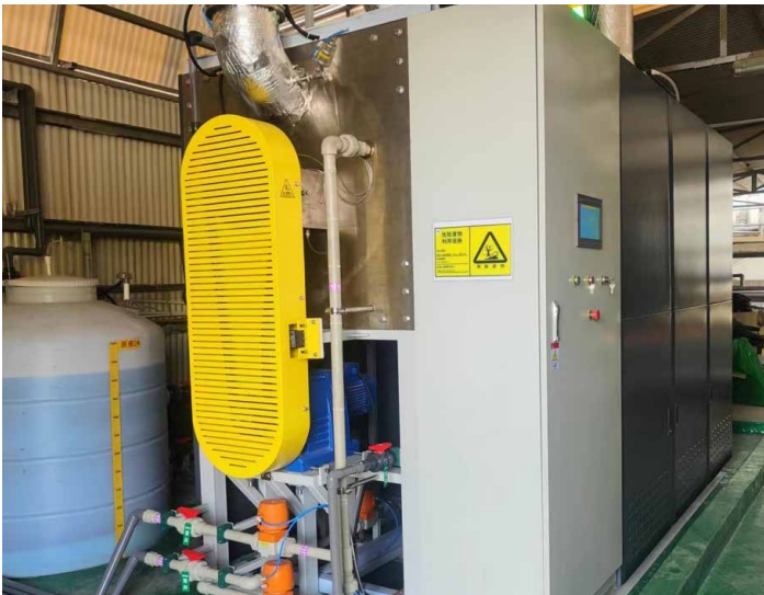
Nickel liquid waste treatment system in TTM Zhongshan
